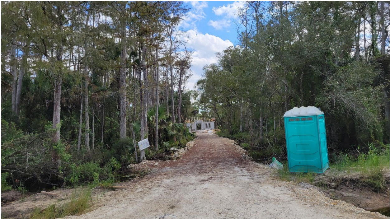
Construction within Horsepen Strand
