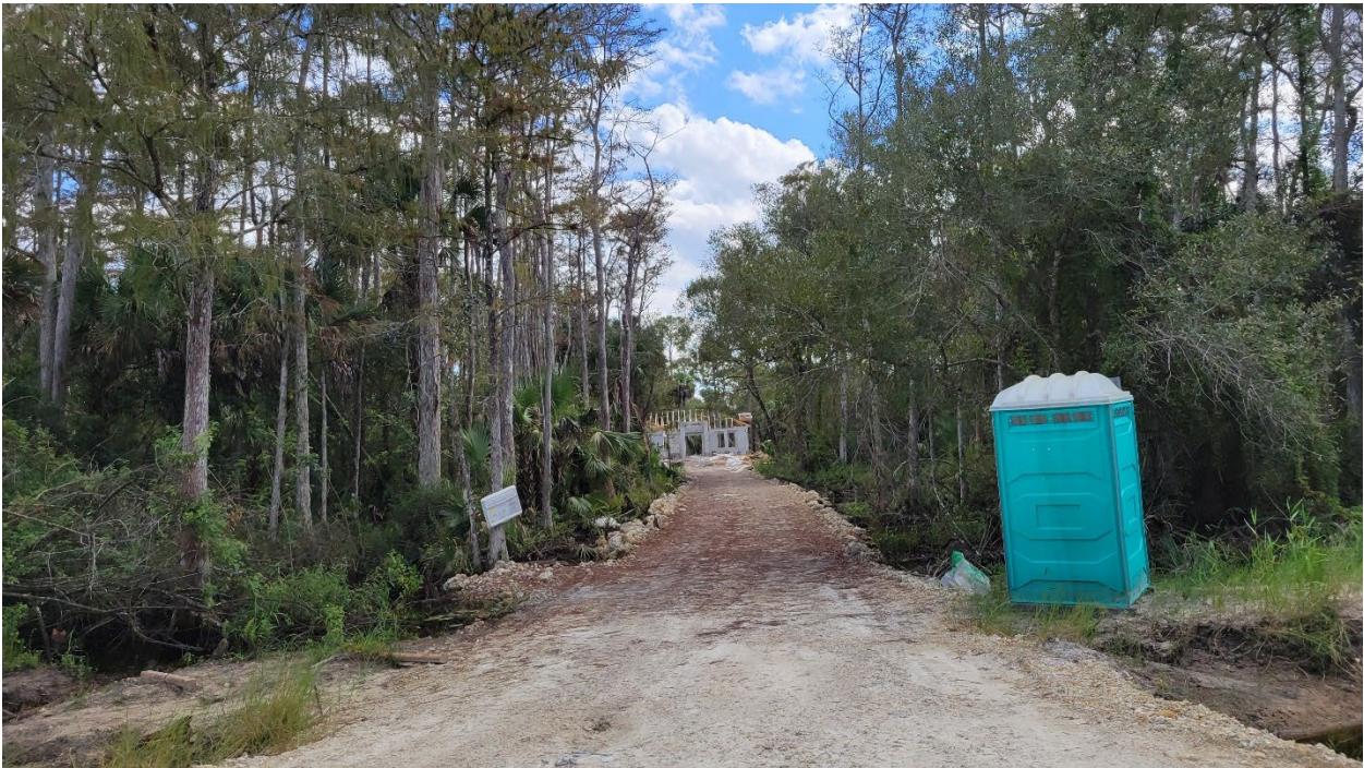
Construction within Horsepen Strand
