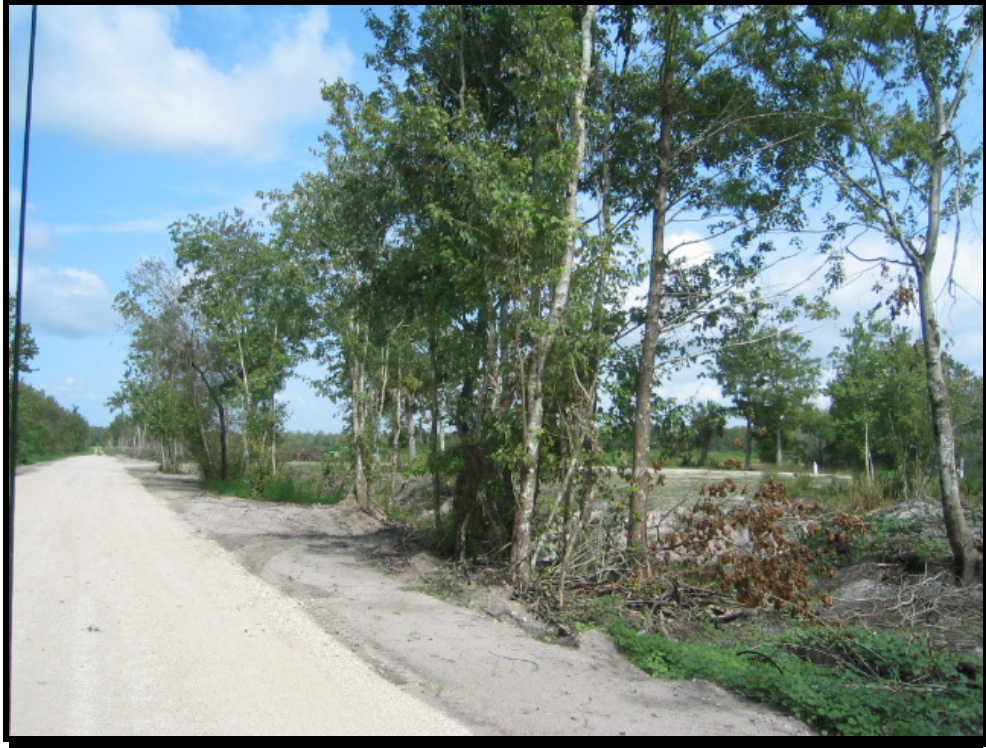
Photo 3. Ditch along Shady Hollow Blvd. (August 2007)
