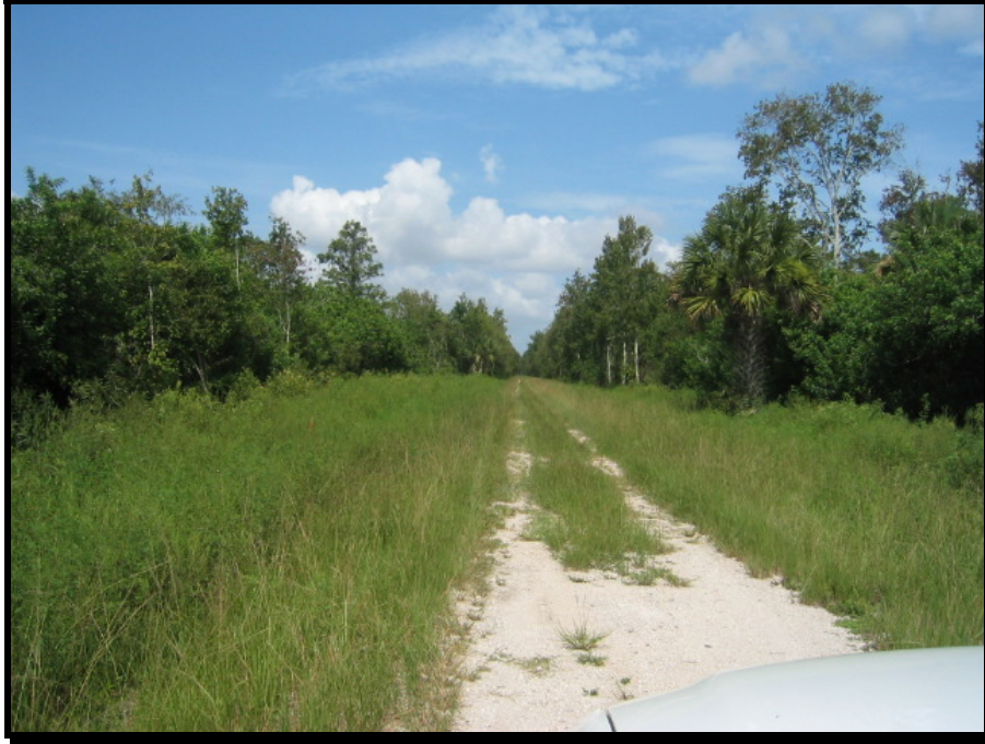
Photo 1. 41 st Avenue NW at the beginning of the east end looking towards the west (August 2007)
