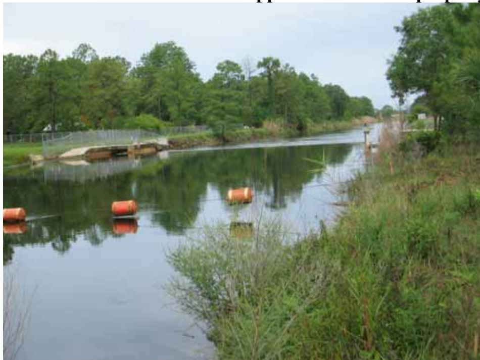
Photo 2. View of canal looking west from southwest corner of property at water control structure in canal – approx. 30 feet from property line
