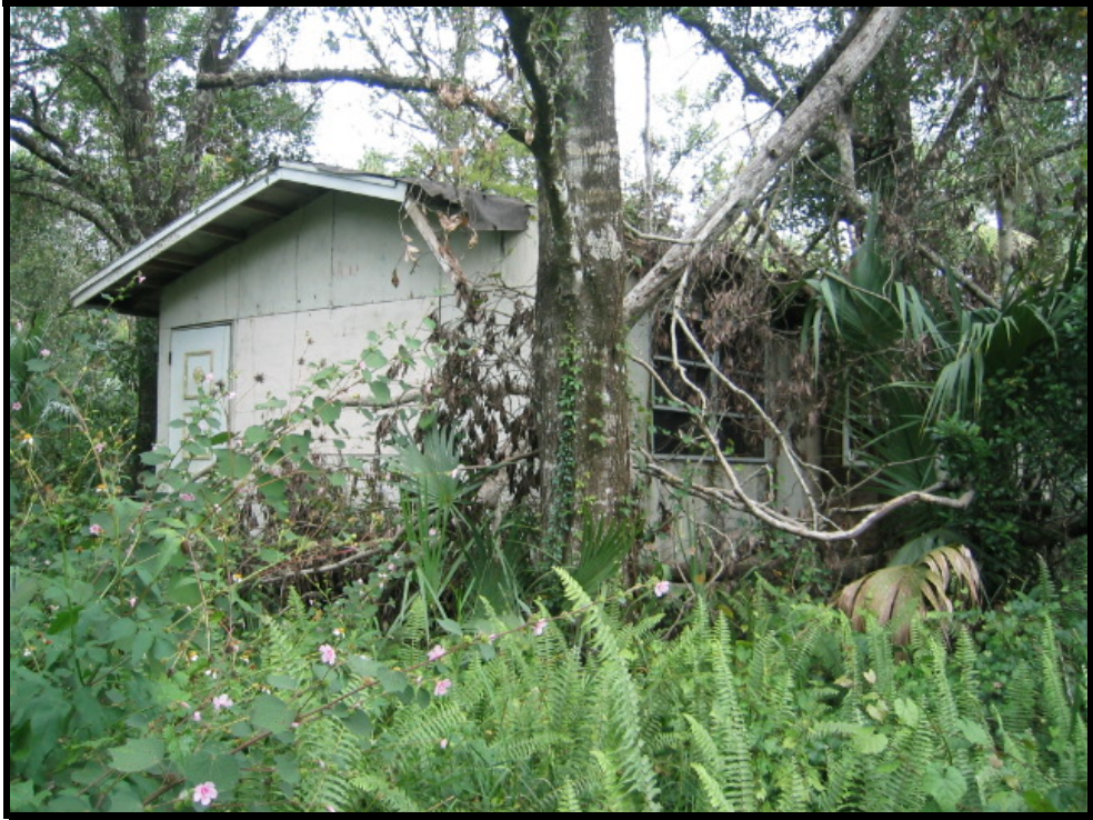
Photo 5. Abandoned house on the property.
