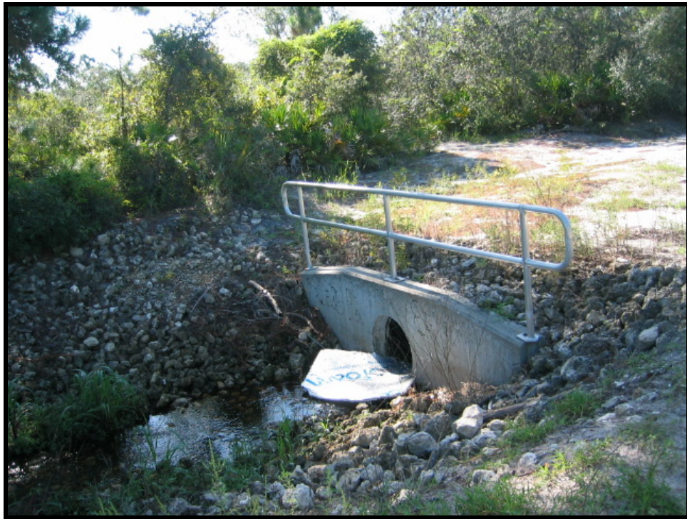
Photo 13. Collier County stormwater drainage structure
