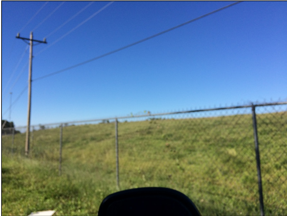
Photo 3. Parcel a. Old Eustis Ave. landfill – south side of Sanitation Road
